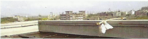
Figure 22. Pipes after replacement with KITEC PE-AL-PE
