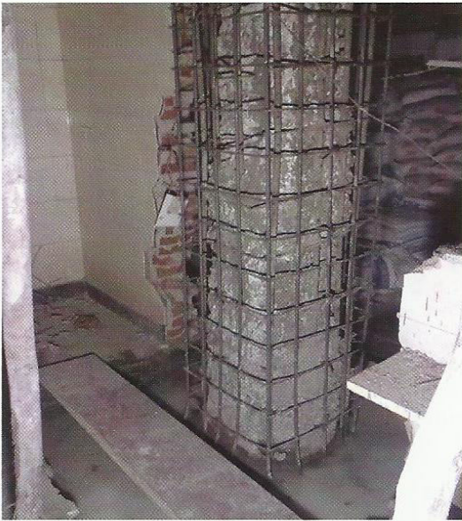
Figure 14. Column before micro concreting
