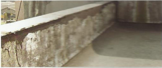
Figure 10. RCC coping before
