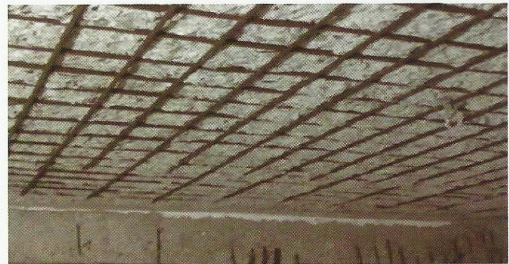
Figure 12. Roof slab before micro concreting
