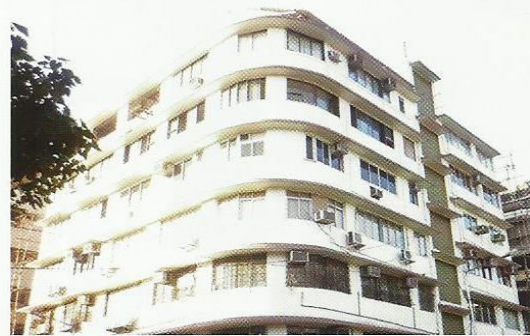
Figure 17. View after coating
