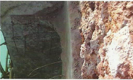
Figure 8. View after breaking non structural elevation
