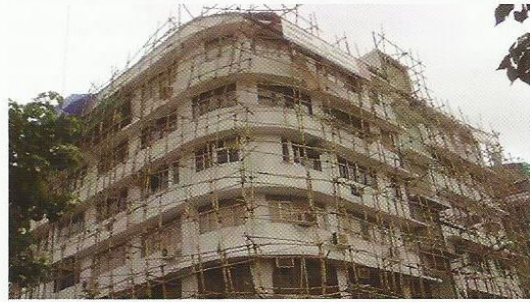
Figure 16. View after primer coat
