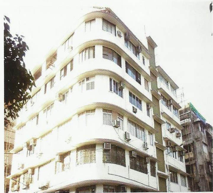
Figure 24. Elevation of the same building after repair and rehabilitation
