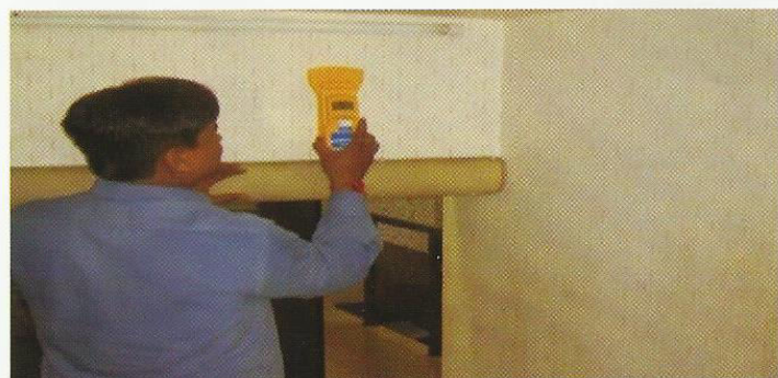
Figure 6. Moisture testing on wall for leakage detection
