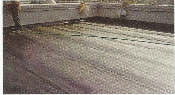
Figure 20. After completion of laying APP membrane on terrace
