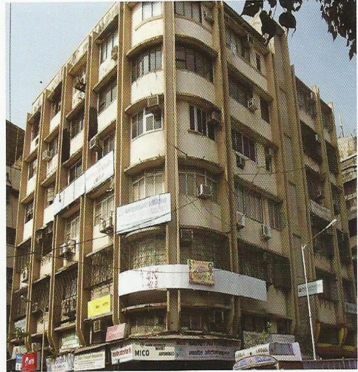
Figure 23. Elevation of the building before repair and rehabilitation
