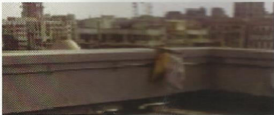
Figure 11. RCC coping after
