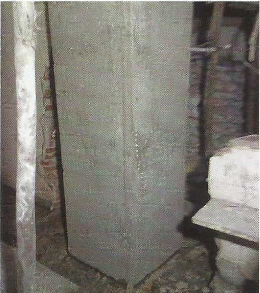
Figure 15. Column after micro concreting
