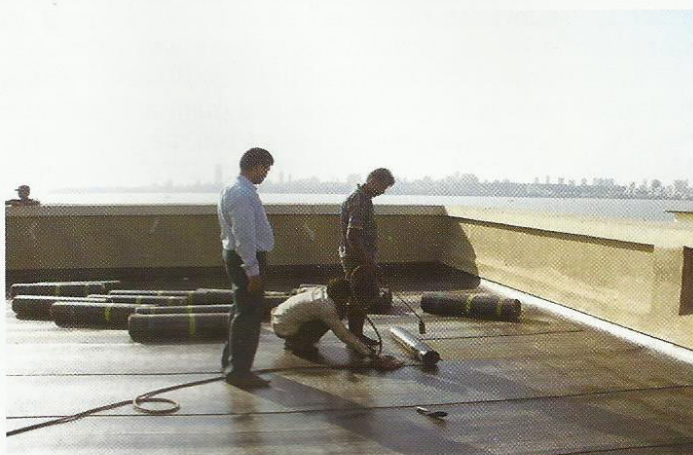
Figure 19. Torch on application of APP membrane for terrace waterproofing
