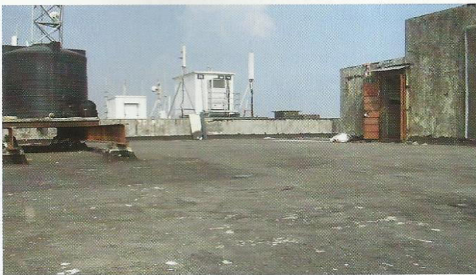
Figure 18. Before roof waterproofing
